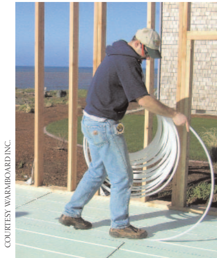
Warmboard radiant heating—installed at the same time as subflooring—combines high-strength tongue-and-groove plywood and APA-rated subfloor paneling with a low mass, high-performance radiant heat floor panel.
