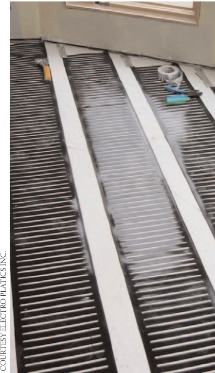
STEP Warmfloor's mat is being installed in this home to create a self-regulating radiant heat system that acts as an efficient on/off sensor.
